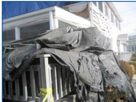
Siding melting off a house.
